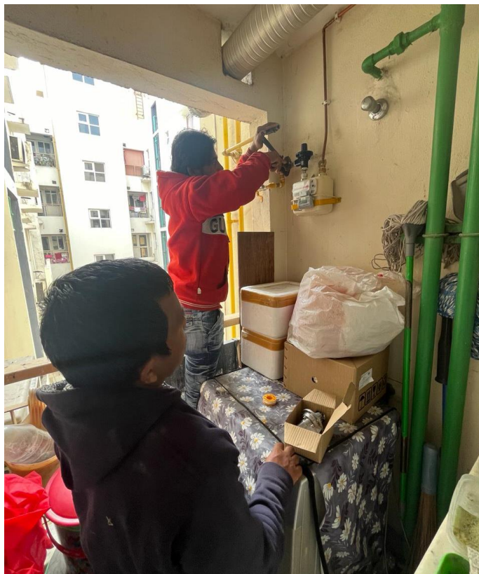
Providing new connection at Housing Societies at Newtown, Kolkata.
